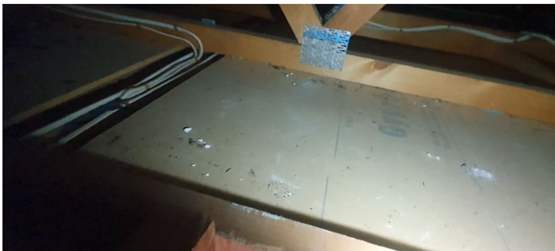
Figure 3.4: No ceiling insulation in a readily accessible ceiling cavity.
