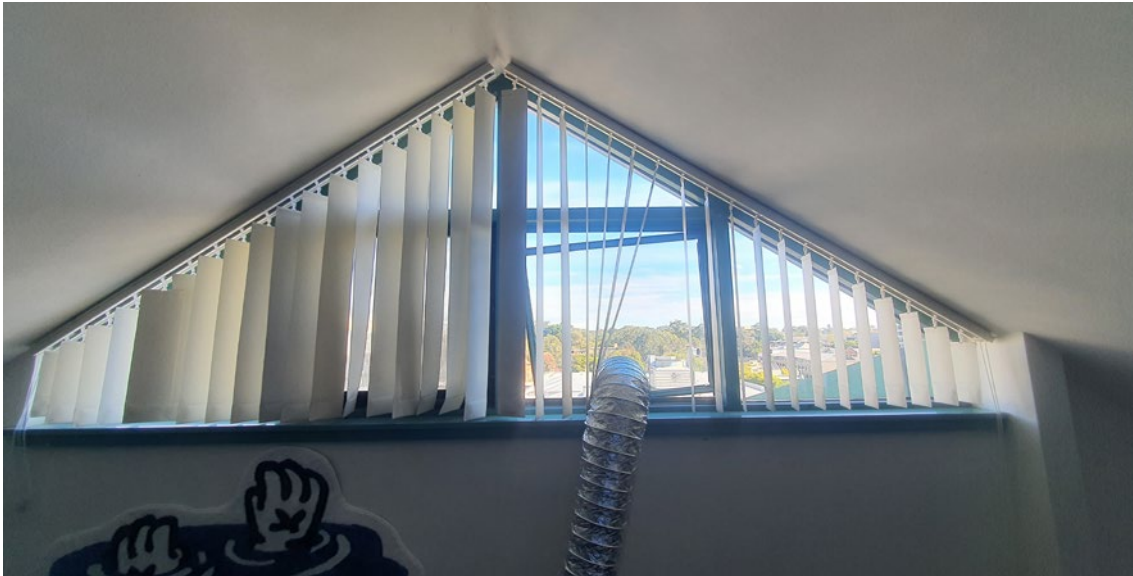
Figure 3.13: Portable air conditioner duct is passed through a broken open window frame with gaps unremediated..
